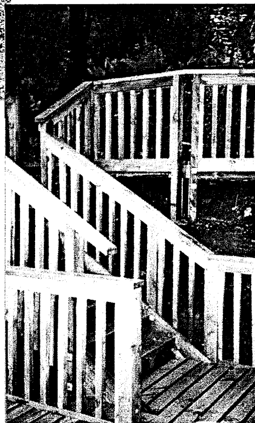
Plate 4 - Infrastructural upgrade at Lake Matheson with new jetty scenic viewpoint (J. Ward).
