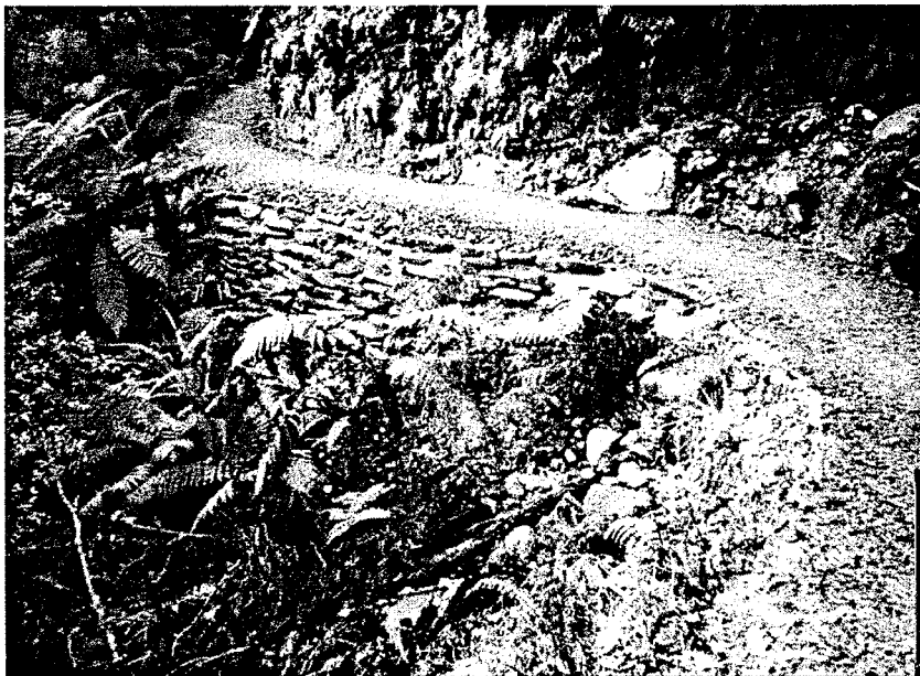
Plate 3 - New hardfill track at Lake Matheson installed in 1999 (DoC Fox Glacier).
