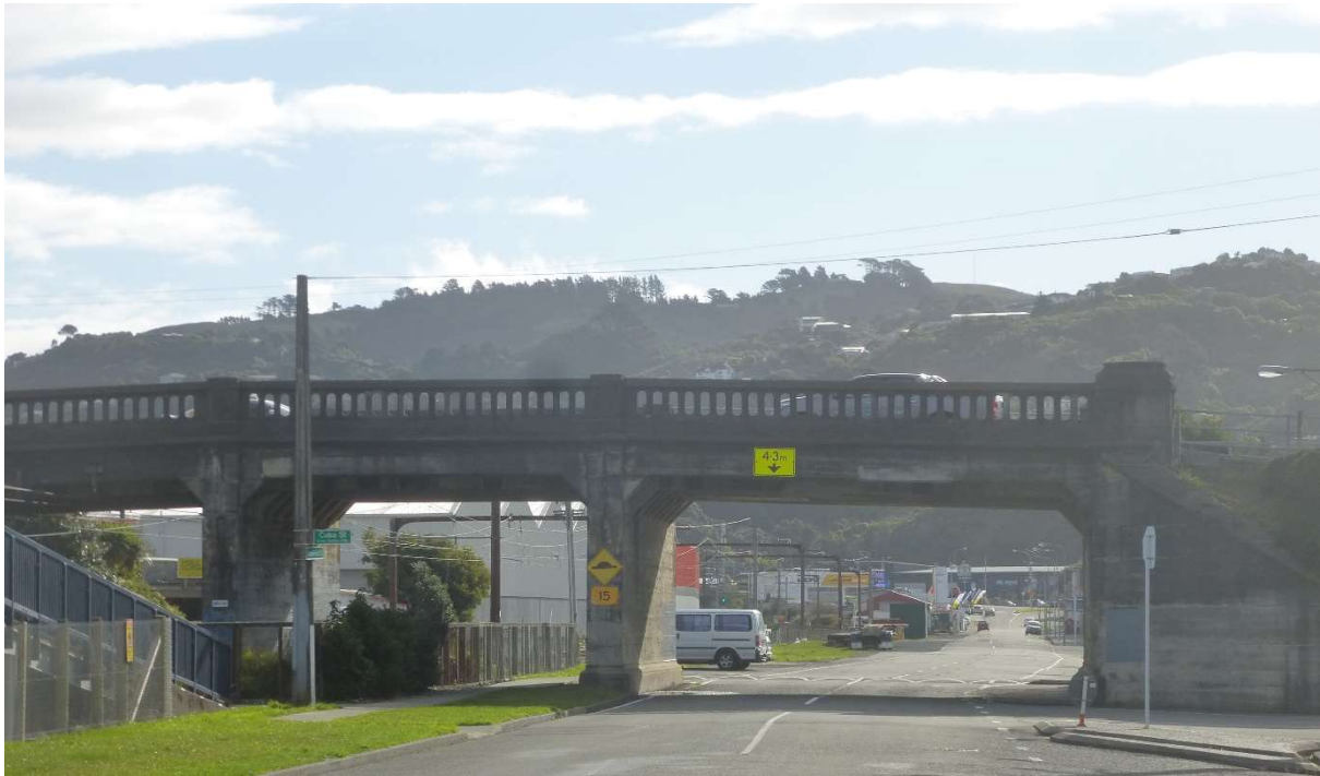
Figure 7: Wakefield st with Cuba street intersecting this area is already part of the inundation zone in Figure 4
