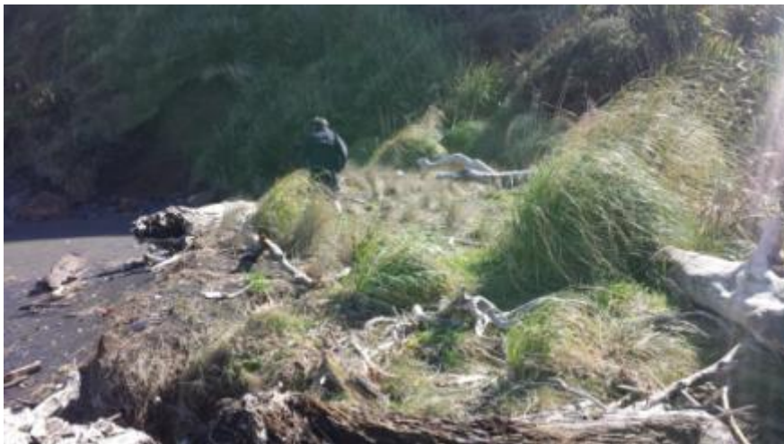
Photo 1: Site inspection 17 September 2014. Overgrown vegetation
