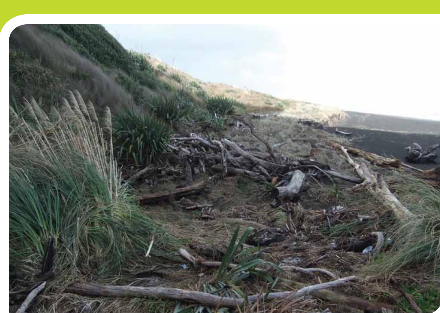
▲ Figure 5-Detection site June 2012 showing surface damage and debris
