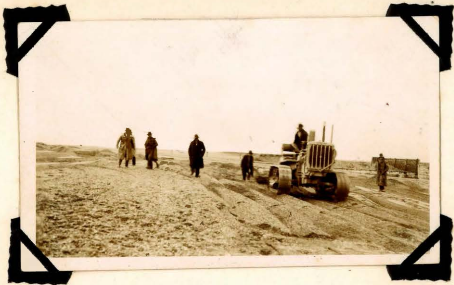
The first tractor used for cutting the pilot channel at Taumutu. In the background is the wooden culvert which had been damaged by high seas and was unusable.
