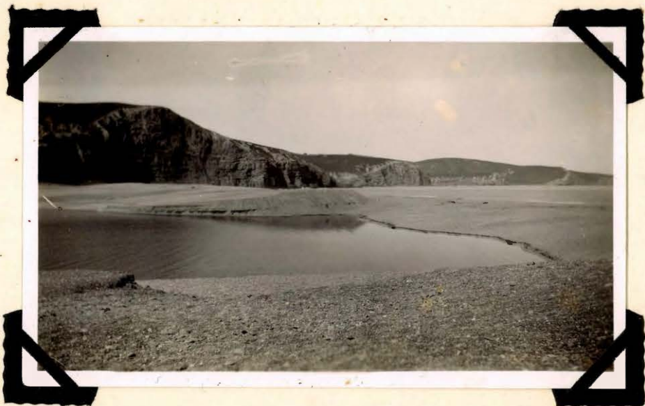
A view of the temporary opening cut through the shingle barrier enclosing Lake Forsyth after it had been blocked by shingle again. The cut through the shingle barrier enclosing Lake Ellesmere is of similar size. In the background are the wave cut cliffs of the Banks Peninsula spurs.
