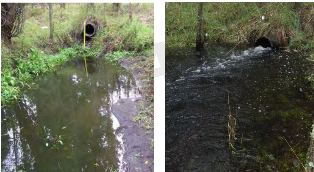
Plates 1 and 2: Culvert One, the culvert closest to the lake on the outlet stream under summer conditions (left, 27 January 2009) and during autumn rain (right, 18 May 2017). The summer photograph is from James and Joy (2009).
