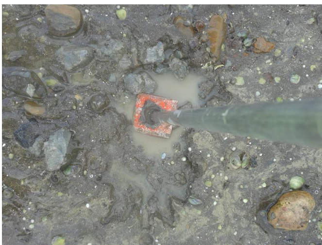
Figure 3.22: Scour around the disturbance rod and seepage collapse at the mid intertidal zone at Moonlight Bay.
