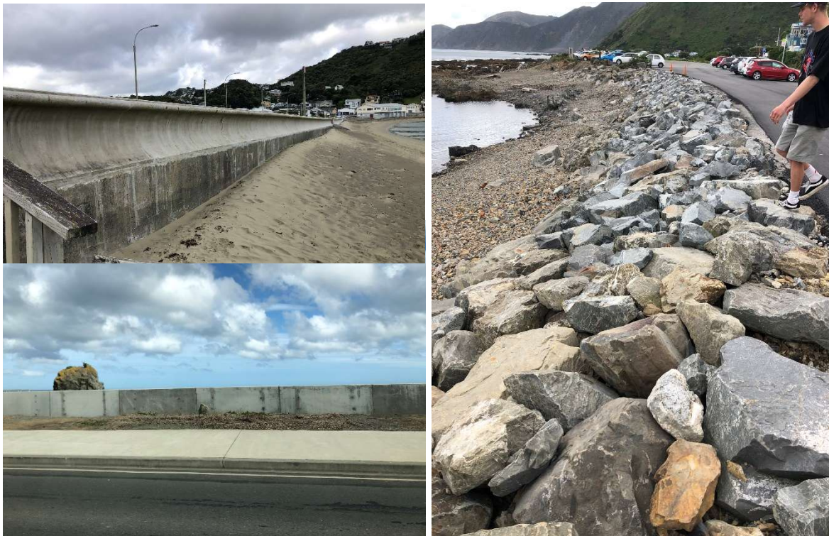
Figure 6.8. Top Left) The re-curved wall at Island Bay. Both Left and Right) The seawall and revetment along the Esplanade near the Victoria University Coastal Ecology Laboratory.
