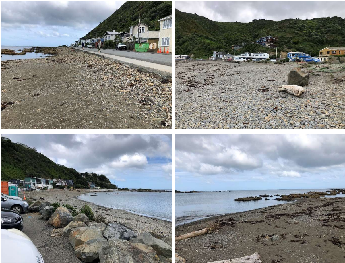
Figure 2.2. Ōwhiro Bay is a shingle pocket beach with platform reefs along the eastern and western sides and is constrained by seawalls and a coastal road around the entire bay (Figure 2.1).
