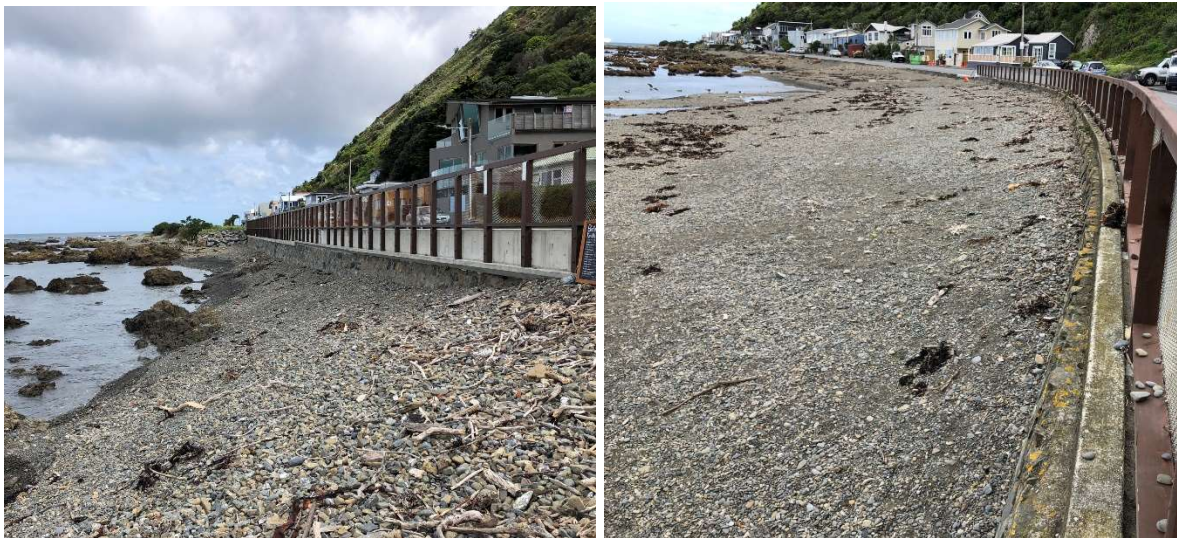
Figure 6.9. The shingle beach is presently almost level with the footpath on the eastern side of the bay where some of the worst over-topping occurred in April 2020.
