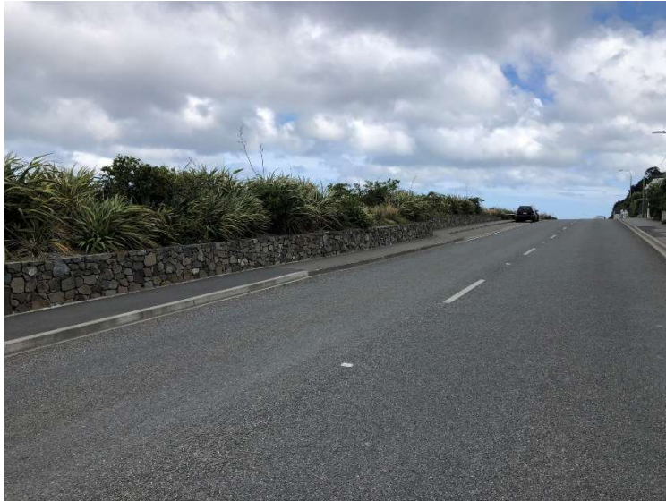
Figure 6.12. A buffer zone of coastal plants along The Esplanade. At Ōwhiro Bay it is envisaged that there would be a lower wall/planting above a graded berm as to reduce any impact on views across the bay.
