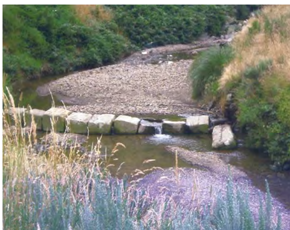
Figure 62: Silt trap at Ngauranga Stream besides Abattoir
