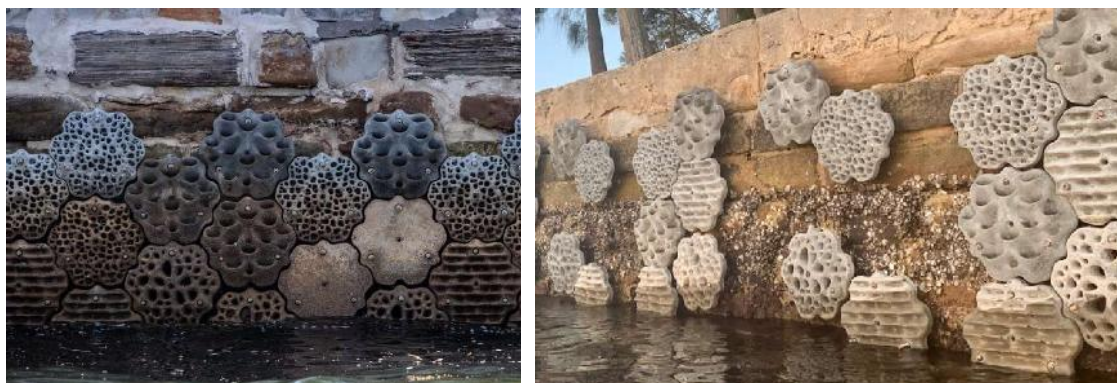
Figure 35: Examples of retrofitted living seawalls.
