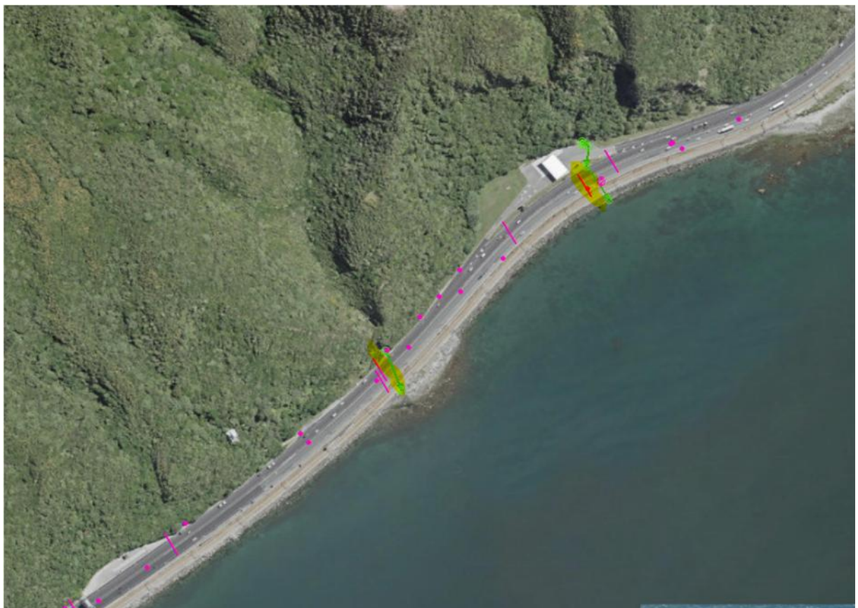
Figure 2: Catchpits and road culverts (Source NZTA)
