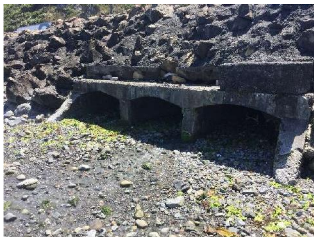
Photo 8: Waihinahina Stream exiting into the coastal environment through culverts under SH2
