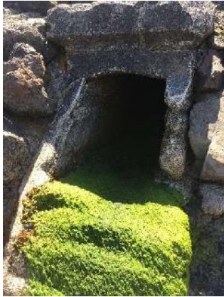
Photo 11: Culvert passing under SH2.
