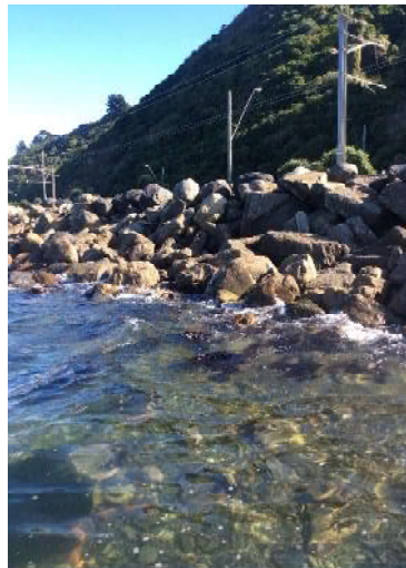
Photo 25: Survey site at chainage 1420m – showing concrete/rock boulder substrate.
