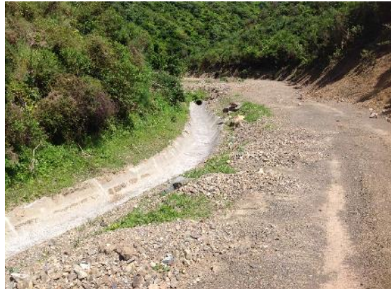
Photo 14: Concrete channel through main gully reach
