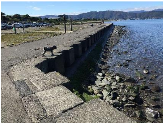
Photo 37: Existing seawall along the eastern coastal margin of the Reserve
