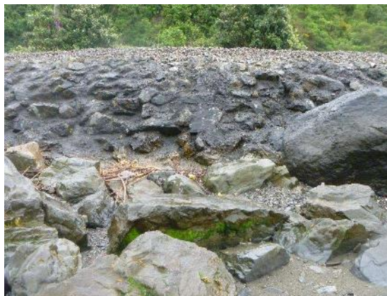
Photo 17: Concrete-rock embedded seawall which provides no crevices for nesting little penguins.
