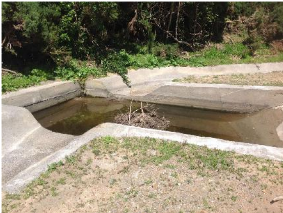
Photo 15: Concrete box settling basin
