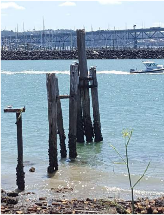
Figure 3: White-fronted terns roosting and nesting on wharf piles at 56 Hamer St
